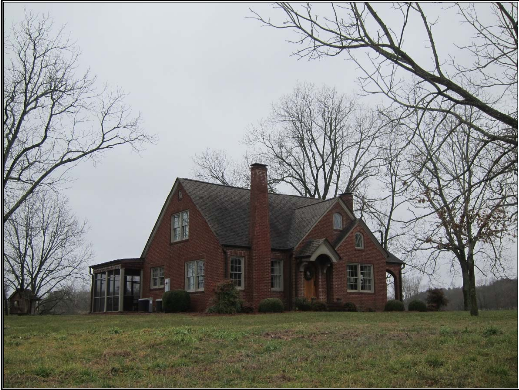
Figure 7. East elevation, facing southwest.
