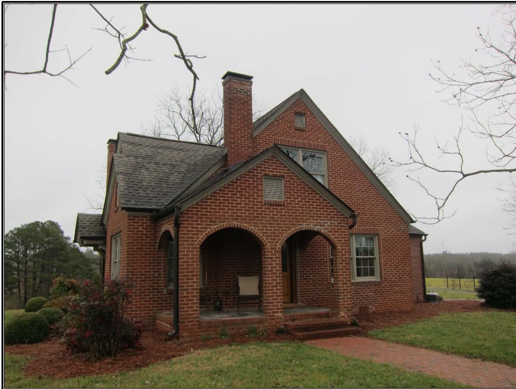
Figure 6. West elevation, facing southeast.
