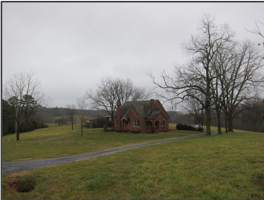
Figure 4. Overview of the Edgar A. Pruett House, facing southeast.
